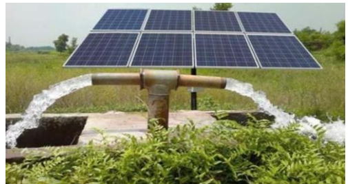
Figure 4. Solar photovoltaic (PV) technology is used to operate a water pump specifically designed for irrigation purposes.
