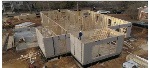
Figure 2 Panelized Prefabrication
