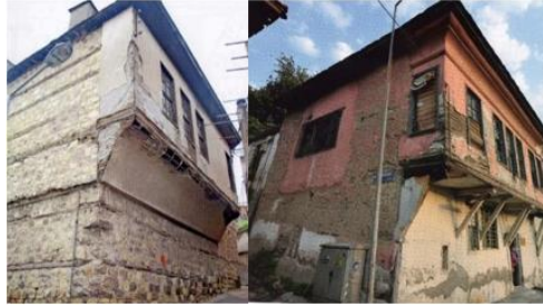
Figure 10. A monolithic masonry wall elevation located on the north face of the housing unit. From left to right, the inventory numbers of the case study houses are 35 and 111 (KUDEB, 2012).
