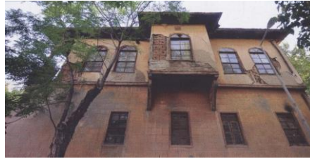
Figure 16. Two-floor Kahramanmaraş house with adobe and timber chock filling on the upper floors. The inventory number of the traditional house is 144.
